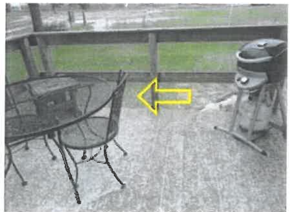
horizontal balusters, open spaces
