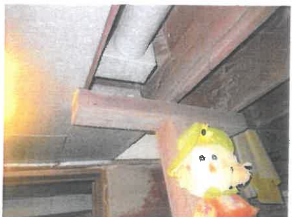
secure post and beam
