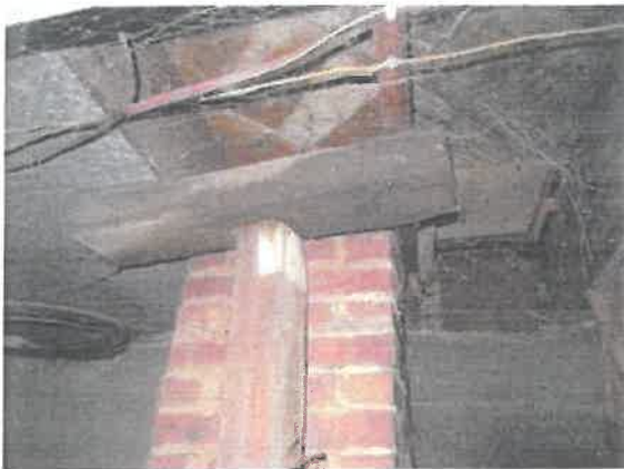
secure post and beam
