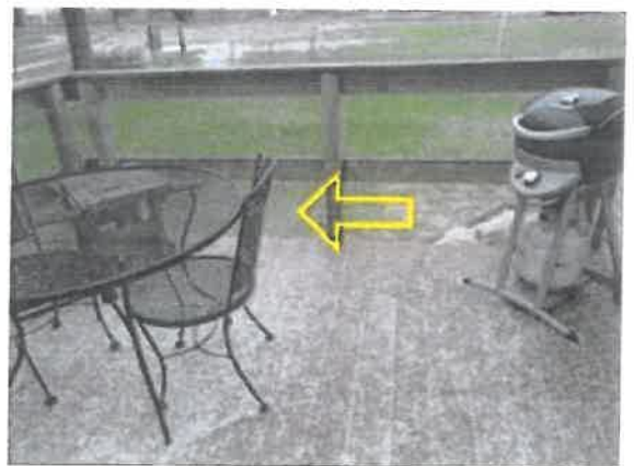
horizontal balusters, open spaces
