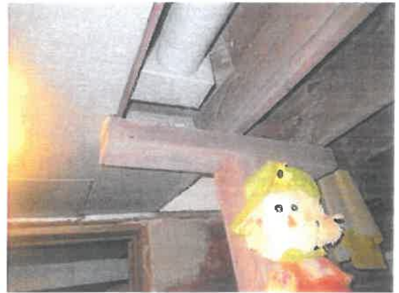
secure post and beam
