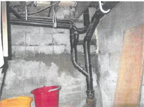
leaking on main
