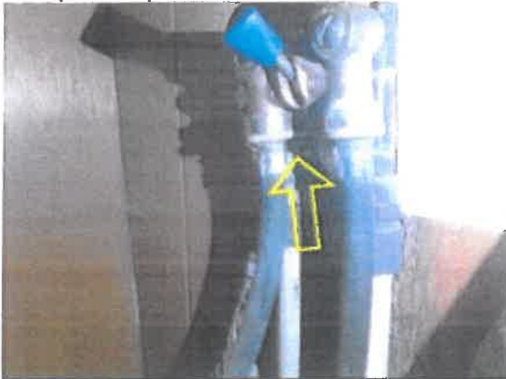
corrosion/leaking
