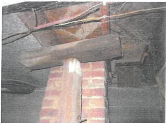
secure post and beam
