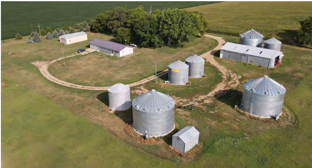
(3) Sioux 20,000 bushel bins all have natural air floors, bin sweep, auger out and were built in 2011 - 2014 - 2016.
