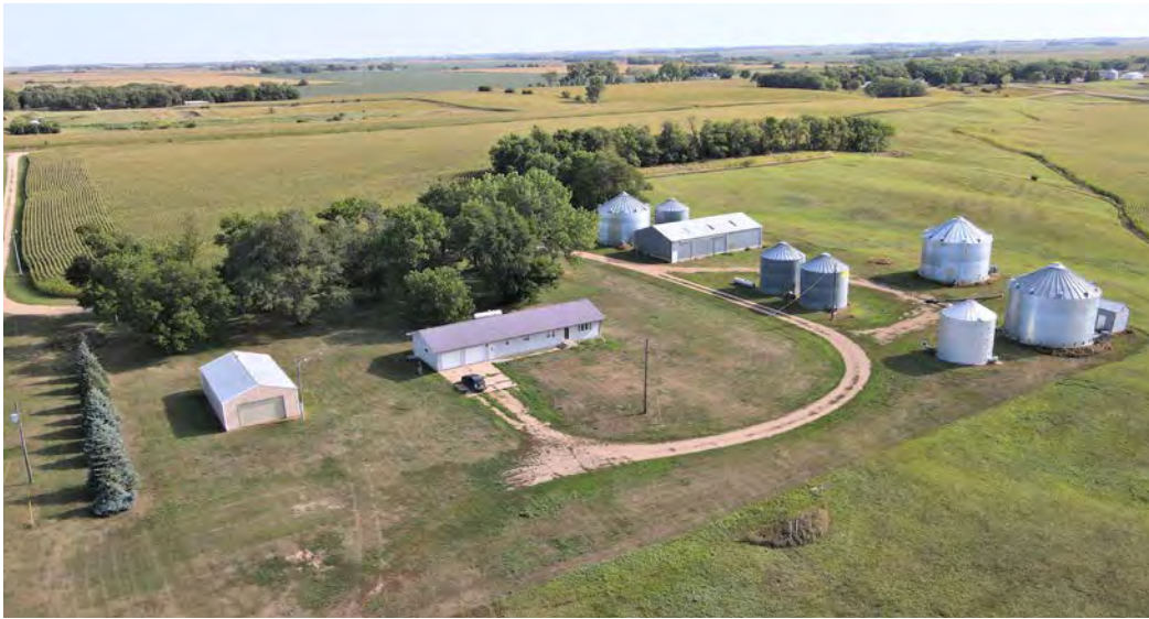
House built in 1983 dimensions 28 x 56 with 28 x 24 two stall garage. 1568 sq ft main floor. 1568 sq ft basement at present all unfinished.
