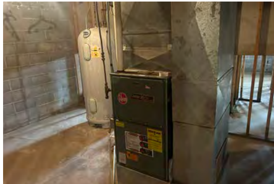
Rheem LP Gas FA Furnace Marathon Electric Water Heater 200 AMP Breaker Panel
