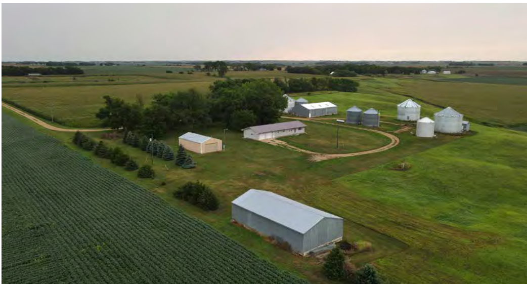
All pole sheds had new poles installed and JRK's attached to old poles in 2024. 40x80 shed has new doors and header on the east side.
